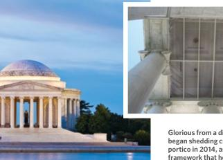
Glorious from a distance, the Jefferson Memorial began shedding chunks of limestone from its portico in 2014, as water corroded the steel framework that holds the ceiling in place. The park service mounted wire netting (above) to catch the falling material—a stopgap until it can afford proper repairs. With nearly a billion dollars in unfunded maintenance on the Mall alone, the National Park Service isn't sure when that day will arrive.
